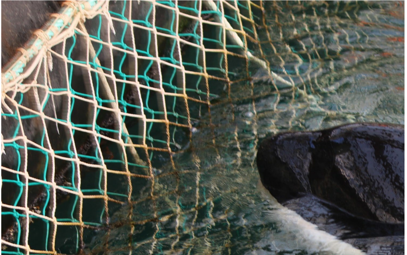
Figure 2. A close-up of an orca next to the mesh netting of its' pen at the Nakhodka facility. This enclosure is constructed (at least in this section) with a 'double internal barrier' comprised of two nets (green and orange/brown) hung into the water. Such double netting will significantly reduce the likelihood that an orca could escape. All three orca pens are also enclosed within a 'barrier net'. (IMG_3697 via Free Russian Whales).
